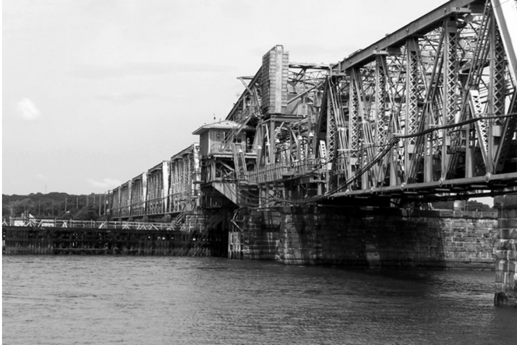
Connecticut River Railroad Bridge, Old Lyme - Old Saybrook, camera facing northwest (HPI photograph).
